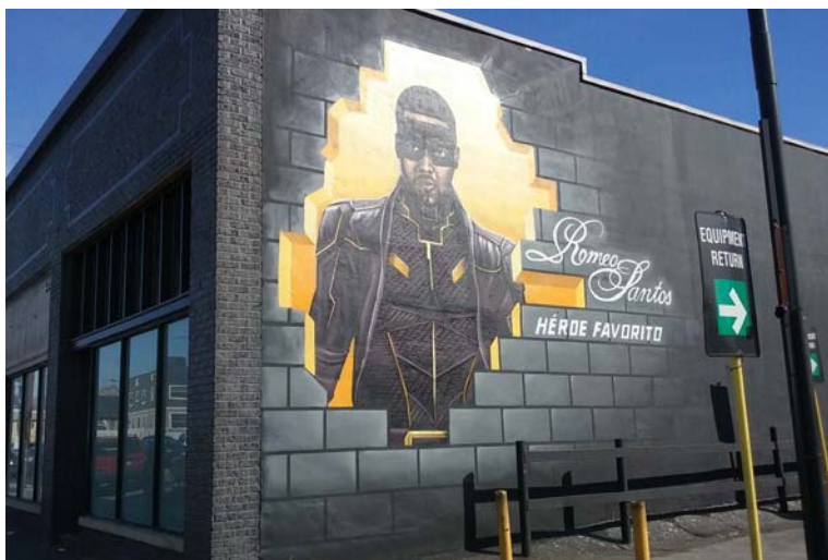
Western Avenue wall, Start Los Angeles building. Photo: Lisa Raymond
